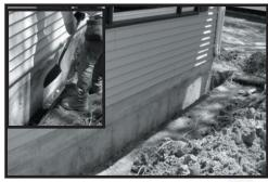
The first step, after contacting your utilities company, is to dig a trench 6" to 12" down along-side the foundation. Seating the panels below grade will help control energy loss.
